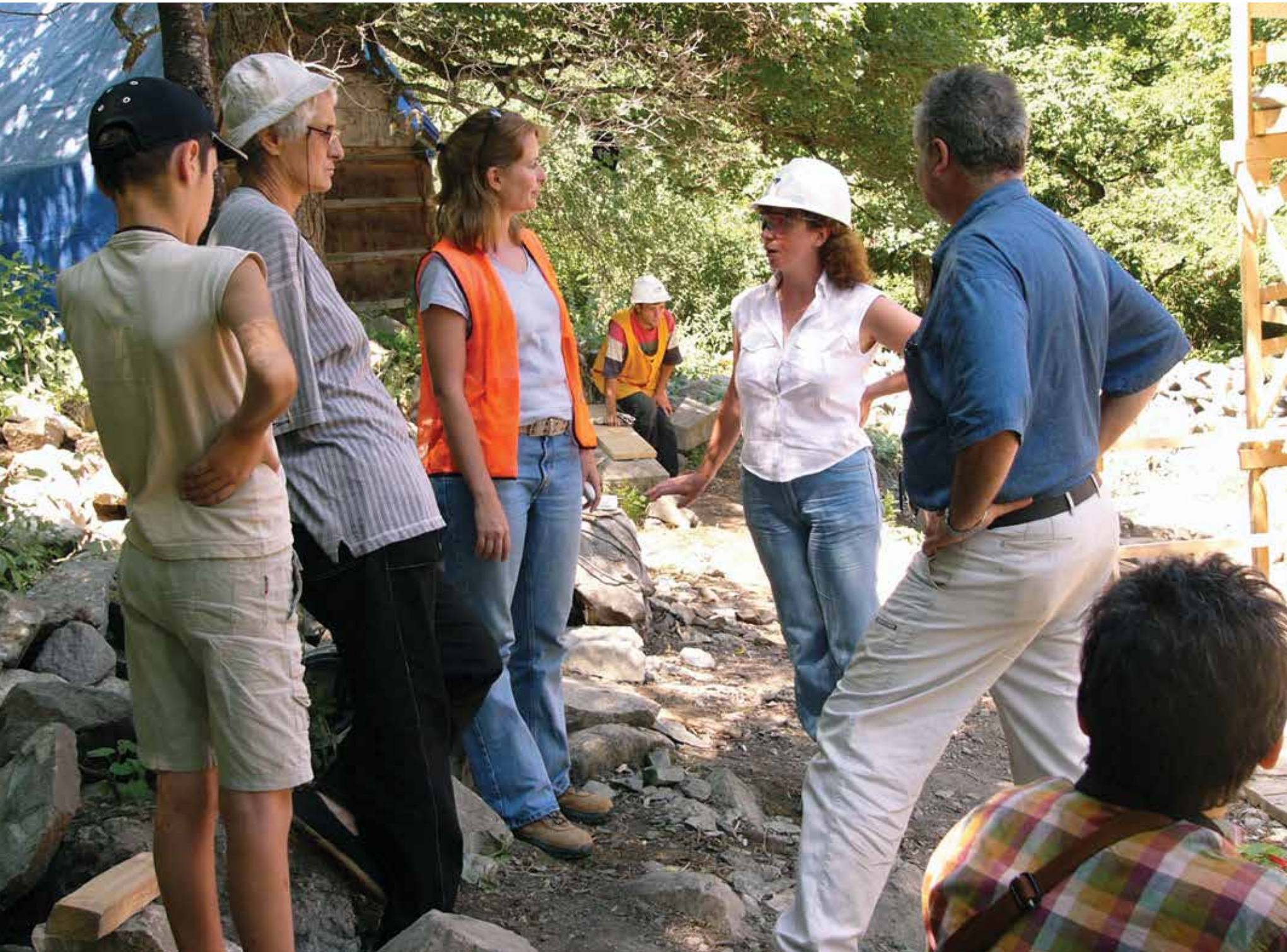
Archaeologist Lali Akhalaia, Cultural Heritage Coordinator Dawn Alexander, Cultural Heritage Monitor Nino Erkomaishvili, and Project Director and Senior Architect Merab Bochoidze discuss the next steps during the restoration of Tadzrisi Monastery in Georgia.
